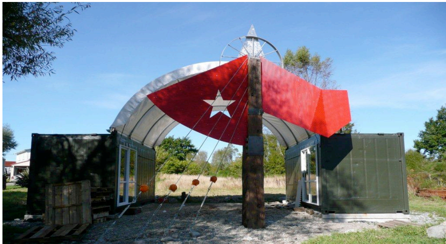
Under construction, Feb, 2010
